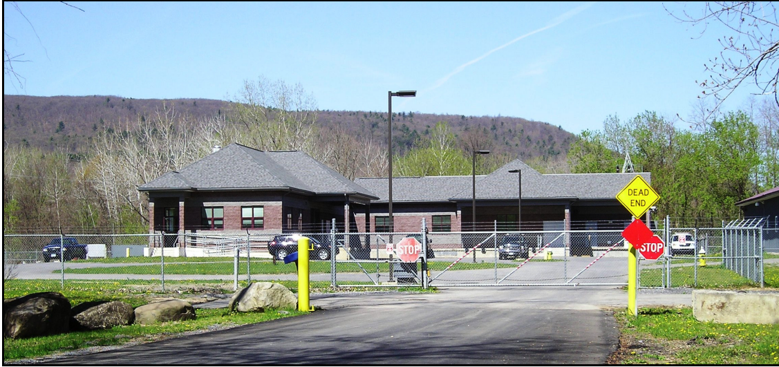
Glenville Water Treatment Plant from Pump House Road
