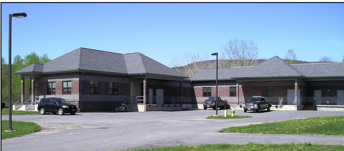
Town of Glenville Water Treatment Plant
